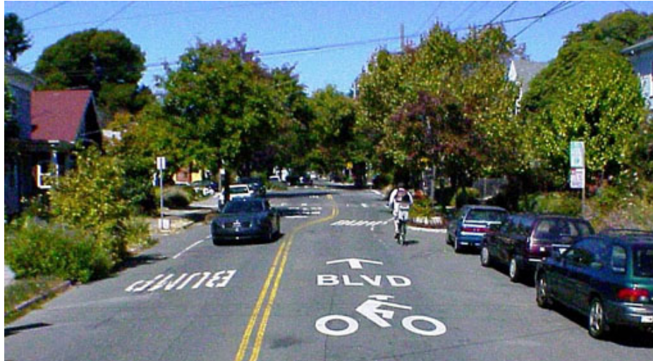
Figure 2—A Bicycle Boulevard in Berkeley, California. Bicycle Boulevards are low-traffic streets which are prioritized for bicyclists. They are a low-cost, highly effective way for a city to immediately integrate bicyclists into its street network. Source: Streetsblog
